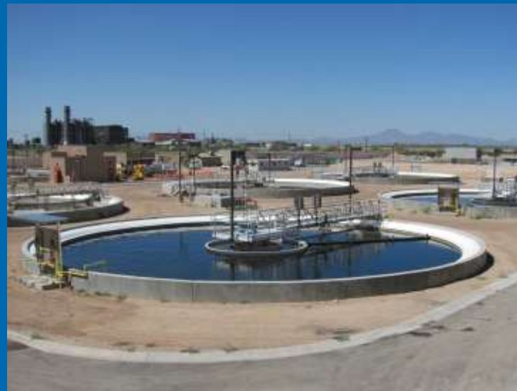
Water Reclamation Facility City of Casa Grande
