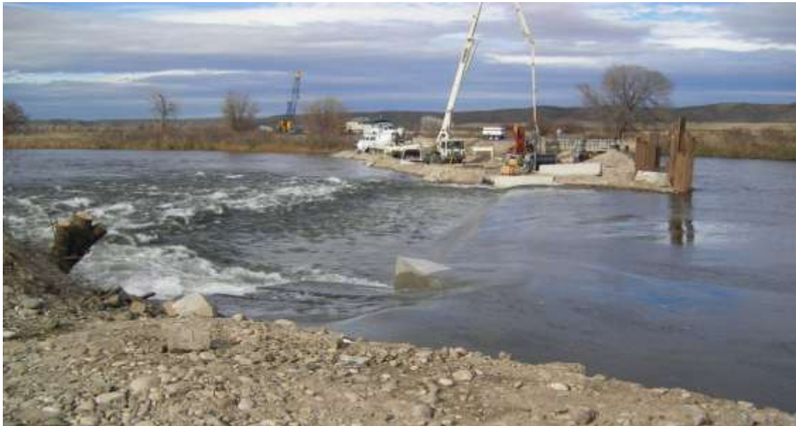
Reconstruction of the Lower Payette diversion structure on the Payette River
