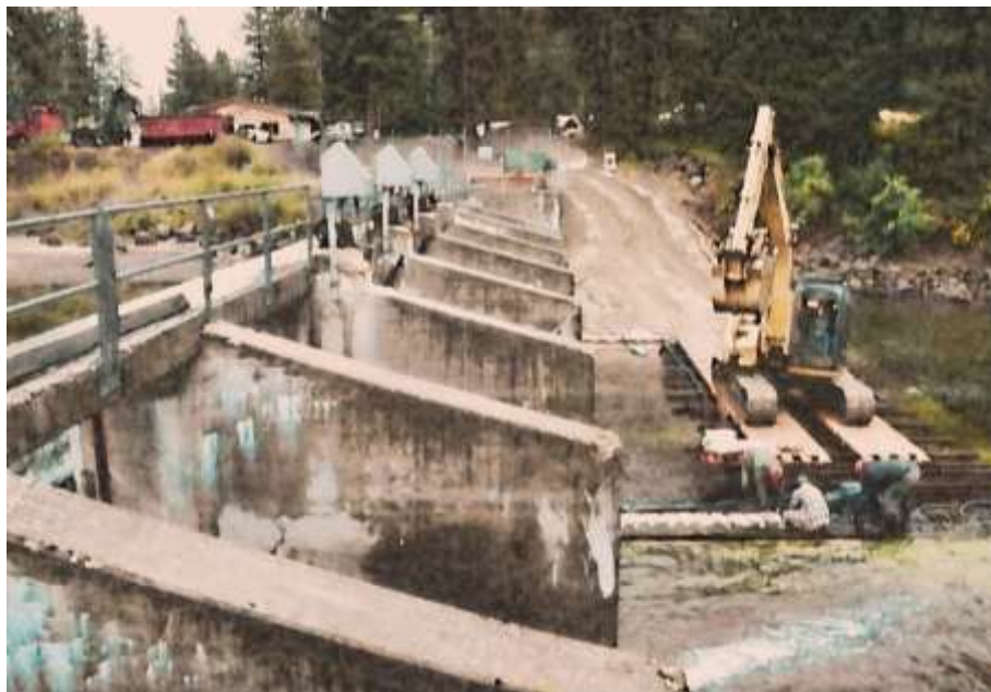
Outlet gate replacement and automation at Payette Lake Dam
