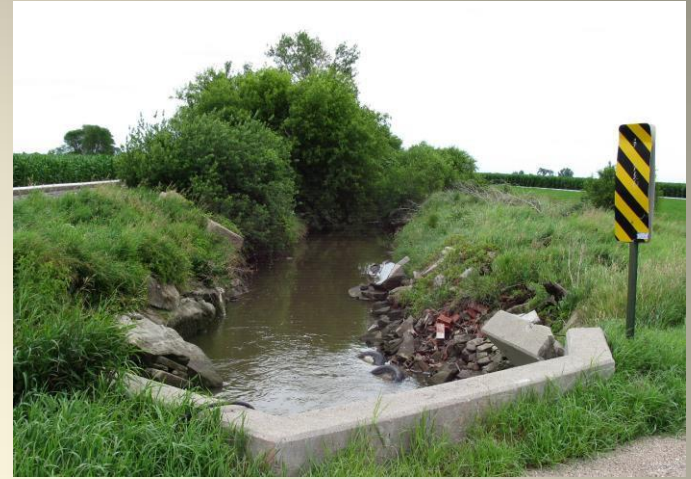
Cozad Canal before clean up.
