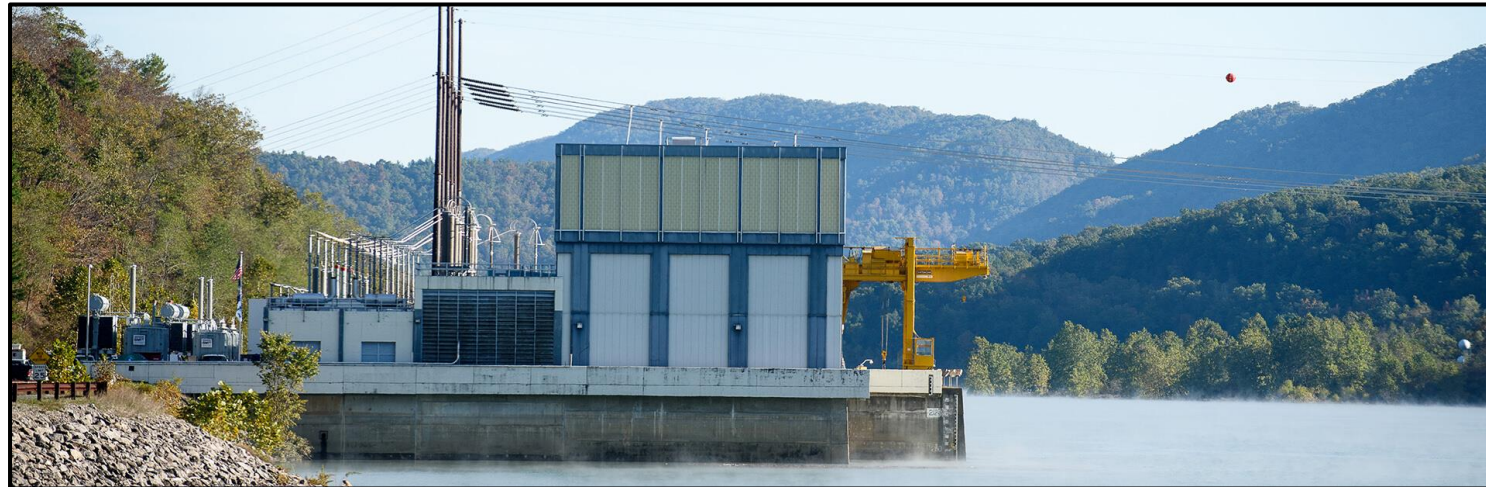
Bath County PSH Project, Virginia
