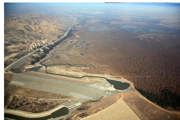
Aerial view of the Prado Dam (Photo courtesy of the Orange County Water District)
